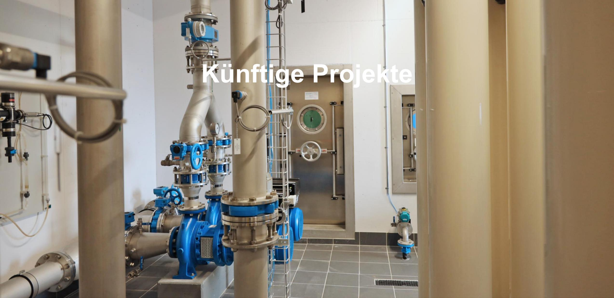
A photograph of an industrial water treatment facility. The scene is dominated by large, vertical stainless steel pipes and complex piping systems. Several bright blue valves and actuators are visible, providing a sharp contrast to the metallic surfaces. In the background, a stainless steel door with a circular window and a handwheel is set into a white wall. The floor is made of dark grey square tiles. The overall environment is clean and well-maintained.
